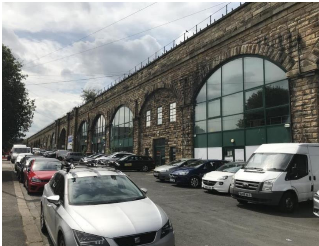
Insert 2-4 Eastern elevation of Huddersfield Viaduct (MVL3/92) on Viaduct Street, showing use of arches by businesses.
