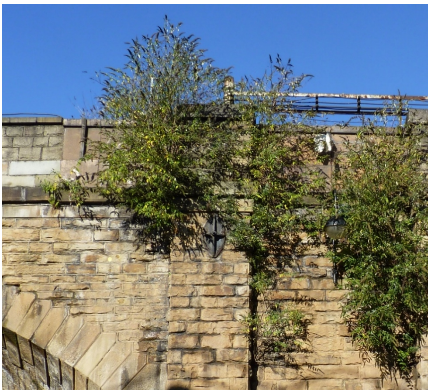
Insert 3-4 Example of existing pattress plate on the eastern elevation of the viaduct, between spans 4 and 5.
