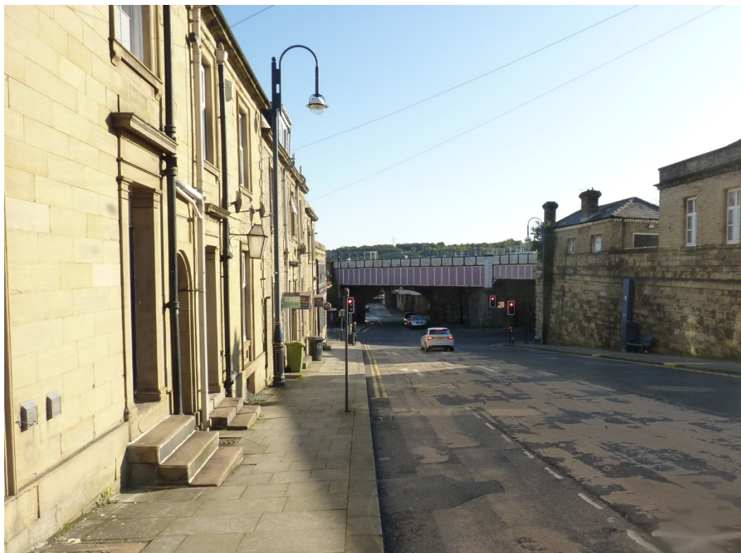
Insert 2-7 View east along Fitzwilliam Street towards Huddersfield Viaduct; note the Grade II Listed 72-78 Fitzwilliam Street (NHLE 1134224) are visible on the left.
