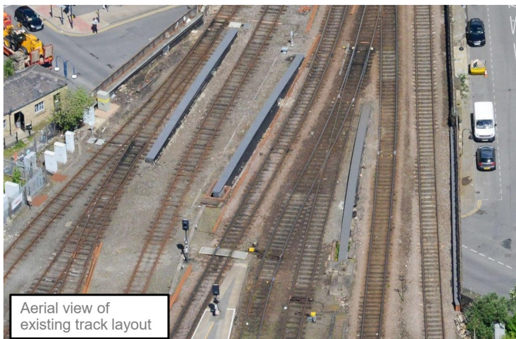
Insert 3-1 Existing track alignment looking north over John William Street (Span 1), showing the through girders of the deck constraining the arrangement.
