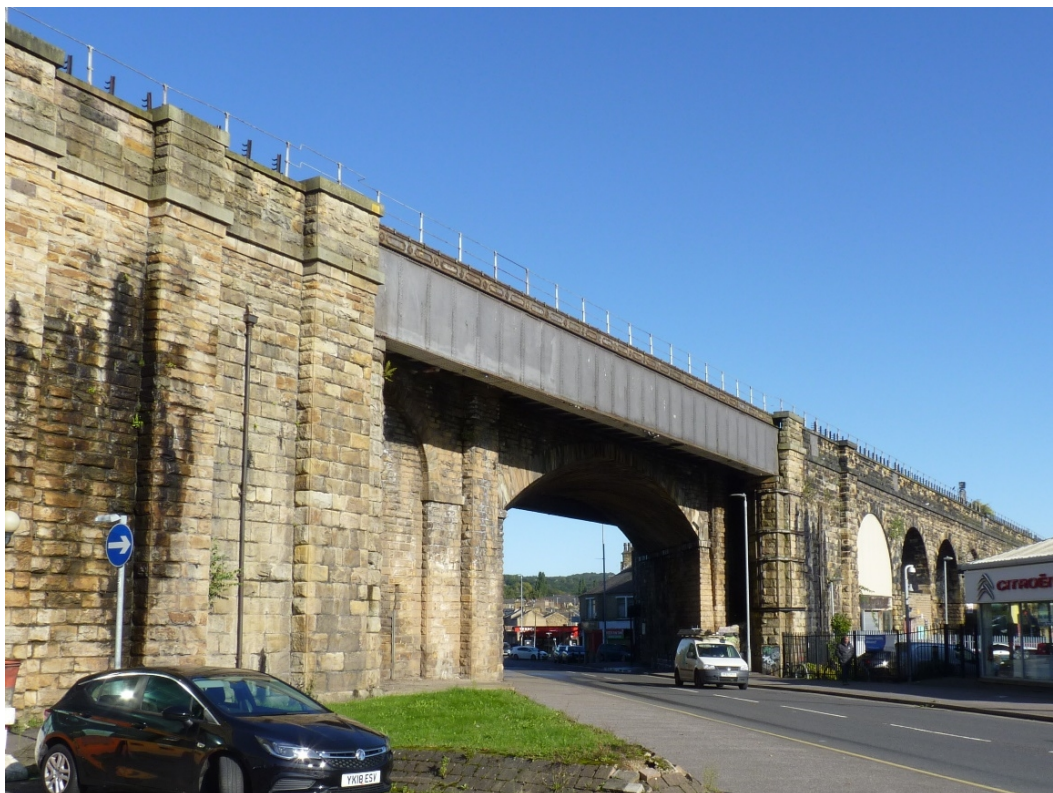
Insert 2-3 Eastern elevation of Huddersfield Viaduct (MVL3/92) , showing 1880s widened metallic span over Northgate / Bradford Road (Span 29), with the original 1840s arch visible in the centre of the span.
