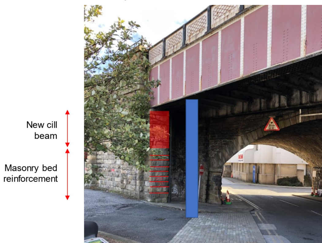
Insert 3-2 Indicative representation of design proposal for works to north-western abutment at Fitzwilliam Street (Span 4) – the blue bar represents the likely temporary propping required during works.
