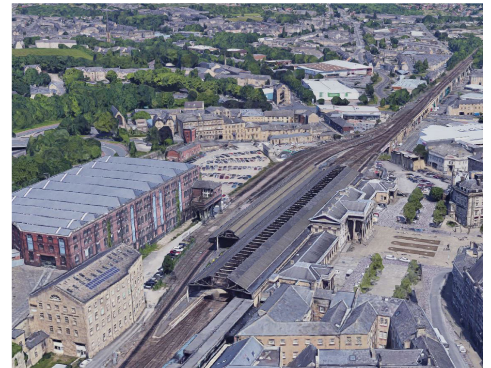
Figure 3.1d: Looking north over Huddersfield viaduct
