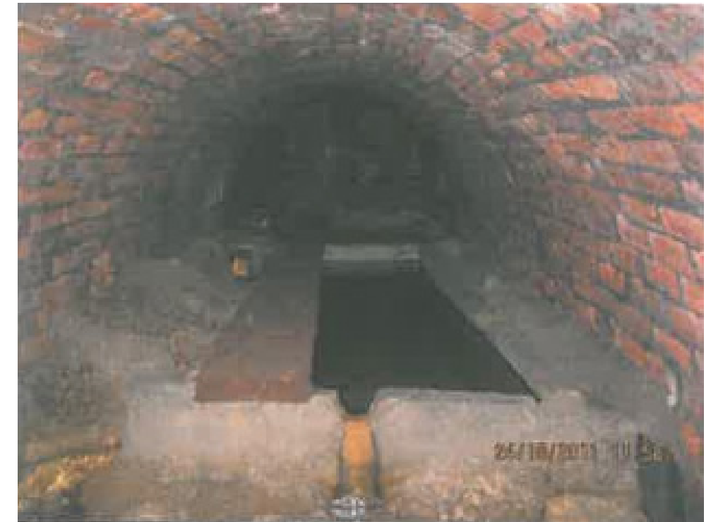
Figure 5.4.8.1b: John William Street culvert
