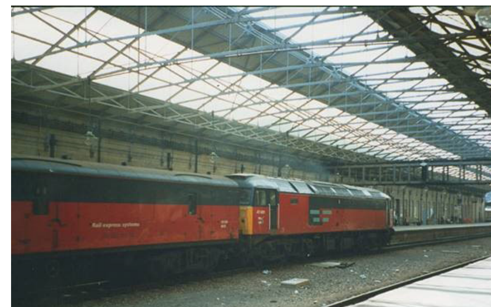
Figure 5.1.6b: Retained Roof A lighting scheme in 1990s
