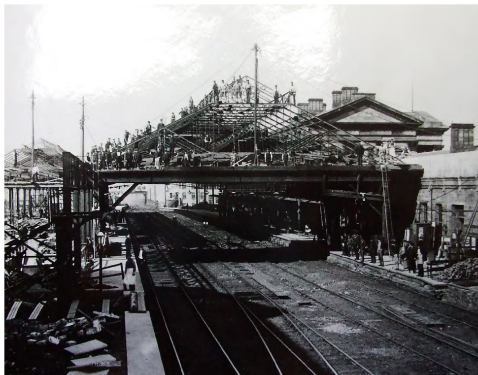
Figure 3.2.3a: Trainsheds under construction 1886
