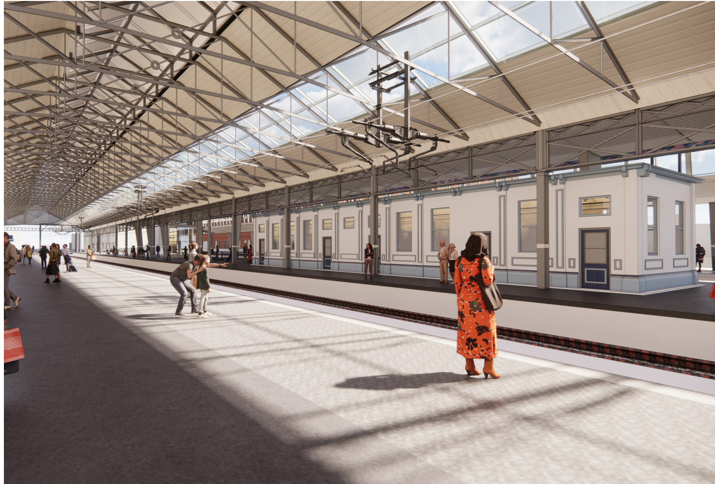
Views through existing Roof A with Tea Room
