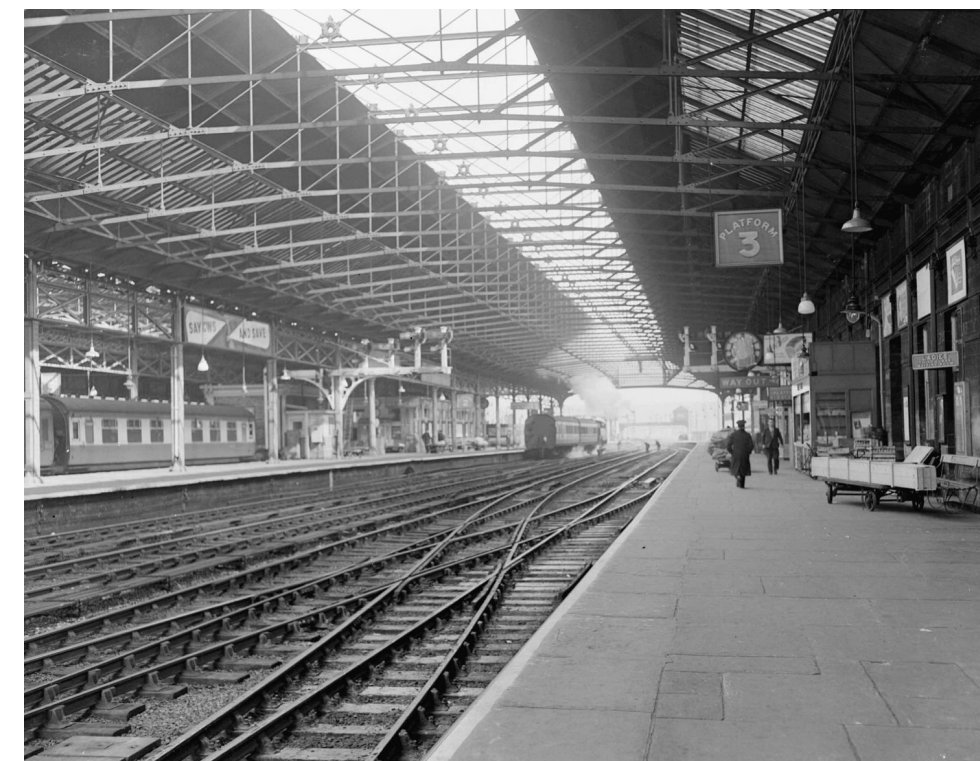
Figure 3.2.3b: Inside trainshed, 1954 with Tea Rooms in distance (The Examiner)
