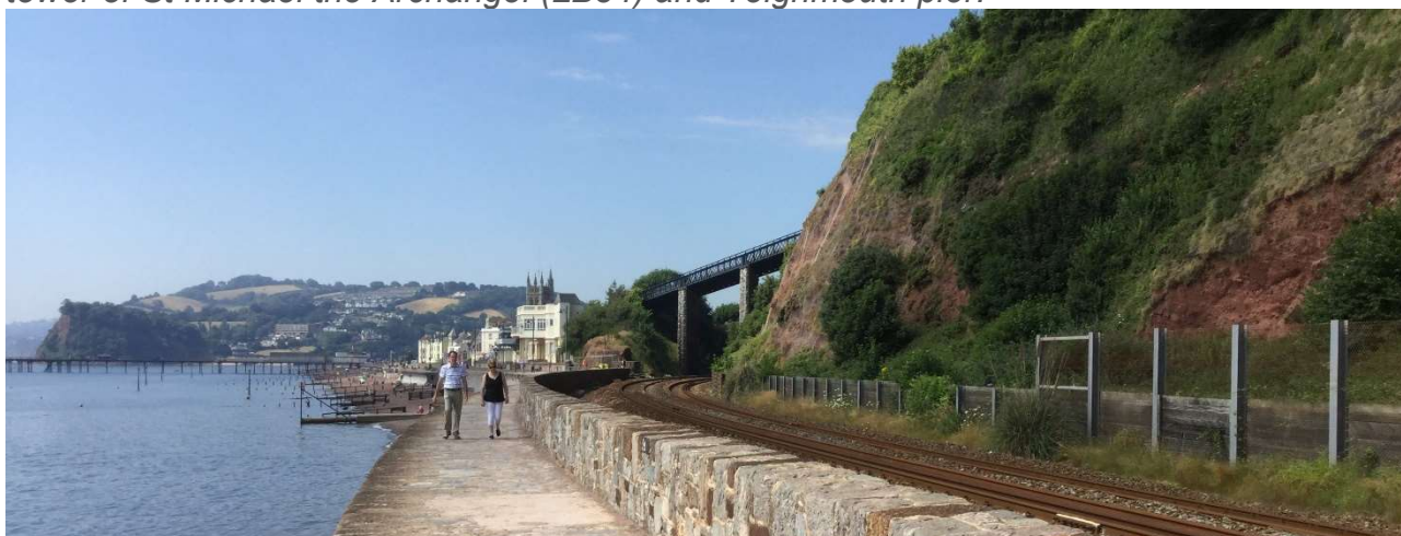
Plate 3 – Looking west from the sea wall at Eastcliff Overbridge (120) showing the tower of St Michael the Archangel (LB34) and Teignmouth pier.
