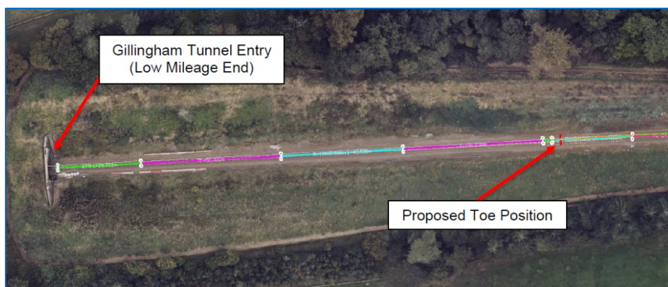
Figure 22: Aerial view of Intervention 2 reverting back to single track prior to Gillingham Tunnel (low mileage end)
