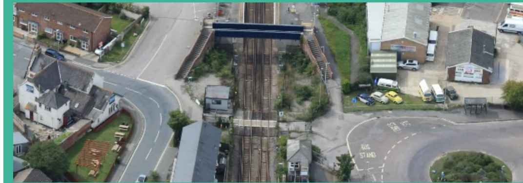
Figure 2: Wareham Level Crossing
