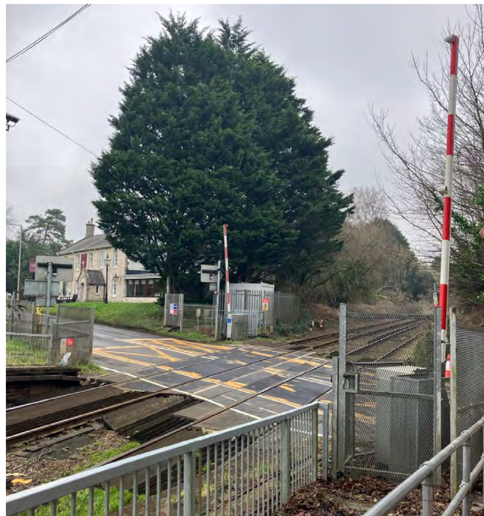
Figure 11: Moreton level crossing, view from platform 2.
