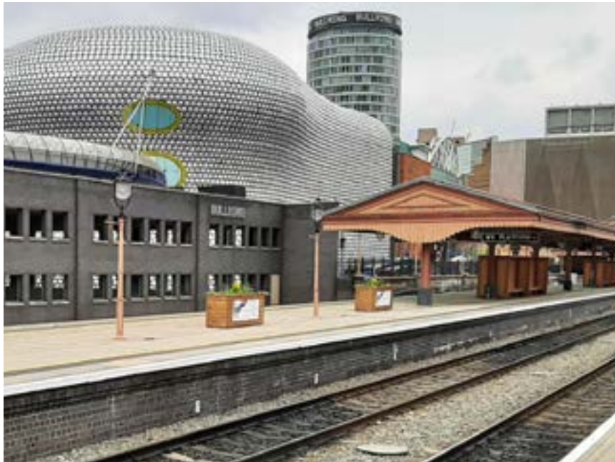
Figure 40: Birmingham Moor Street Station, a key component of Midlands Rail Hub
