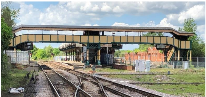
Figure 24. March station (looking towards Peterborough). If a passenger rail link to Wisbech is re-established, it could potentially use one of the disused platforms on the right.
