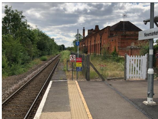
Figure 34. Newmarket platform – the current four-car length of usable platform will require extending to accommodate through services
