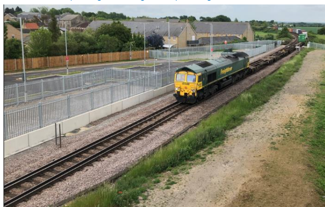
Figure 4. Soham. Northbound F2MN freight train entering the single-line section between Soham and Ely.
