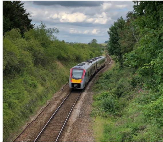
Figure 5. The Newmarket single-track section. The line was built as double track – except for the section through Warren Hill tunnel (Newmarket).
