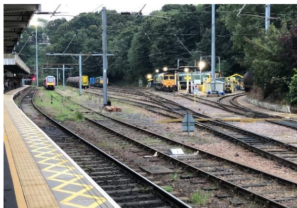
Figure 8. Freightliner fuelling point at Ipswich. This facility has now been relocated. New platforms 5 and 6 could be located on the site
