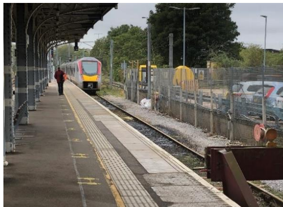
Figure 7. Ipswich platform 1. An additional track and a new platform 0 could be accommodated alongside. n.b., the position of the stationary train is due to platform 1 not being electrified for its full length – see section C.8.
