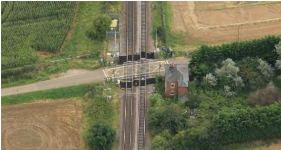
Figure 10: Rowston level crossing, between Sleaford and Lincoln
