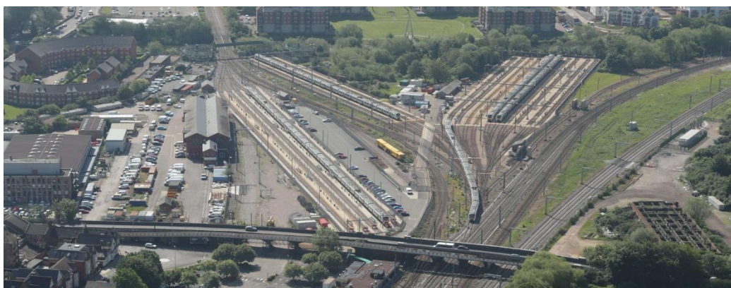
Photo: Bedford sidings – Network Rail
