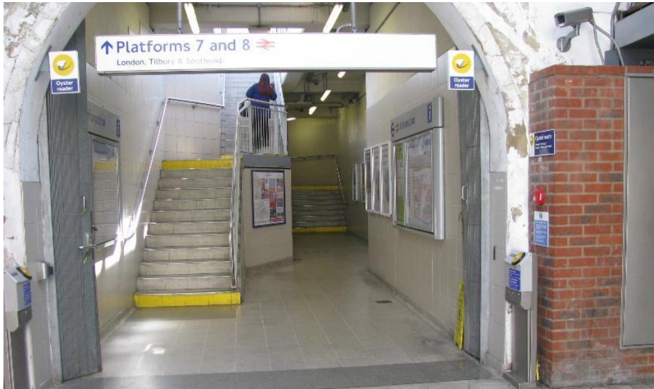
Figure 19 – Narrow stair access to West Ham’s National Rail platforms. A lift is situated behind the nearest staircase.
