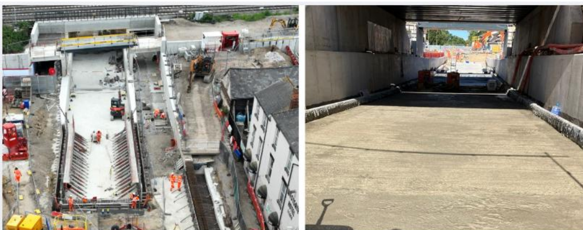
Pictured above: new ground water flood defence structure completed.
