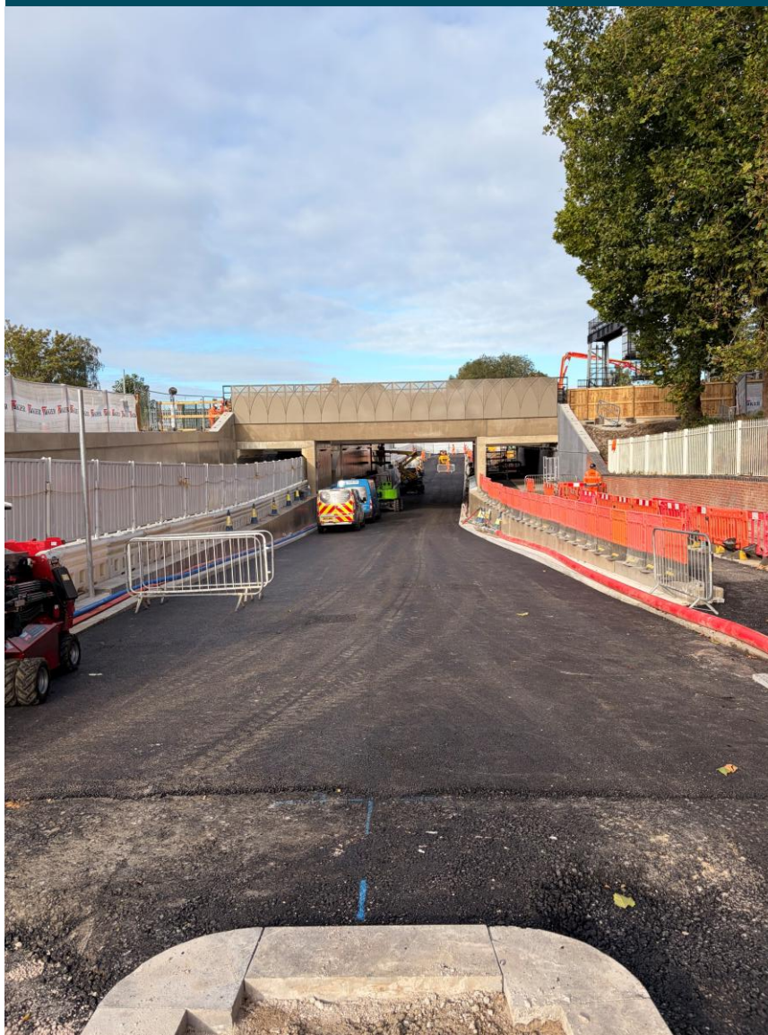
Botley Road looking west and east
