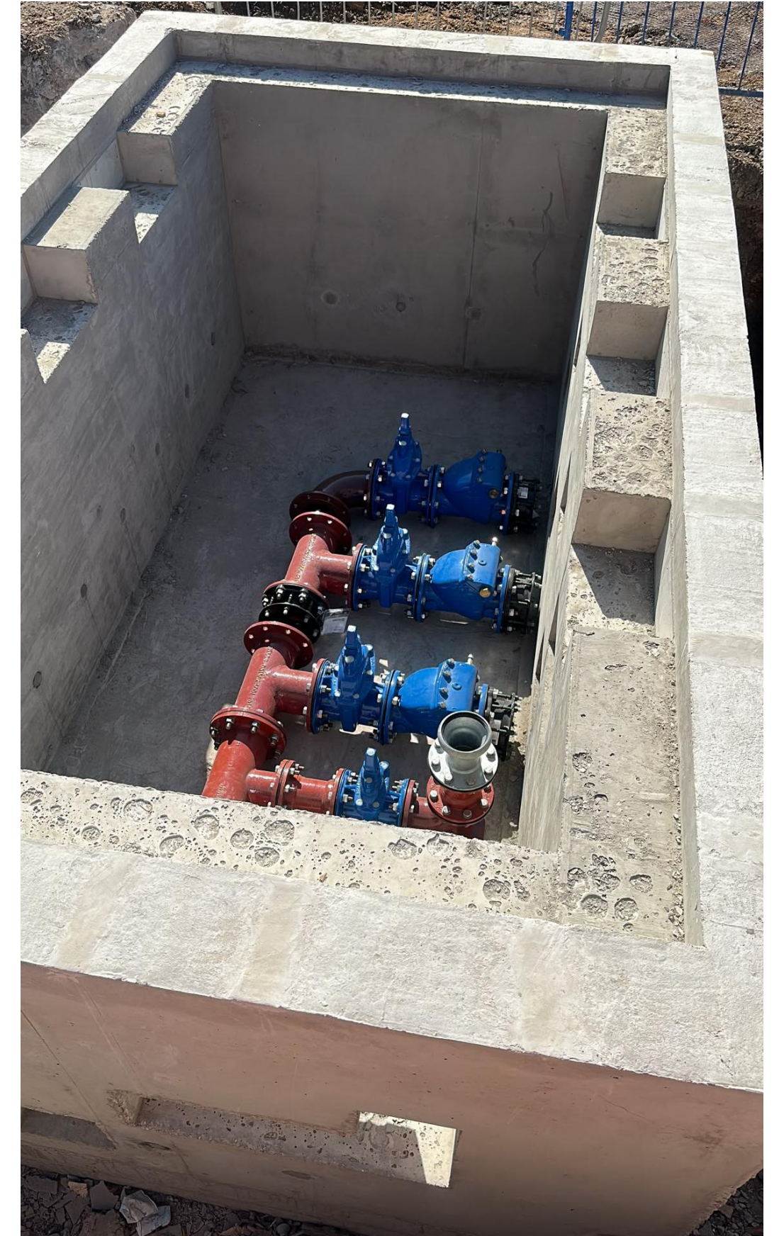
Right: valves installed in chamber
