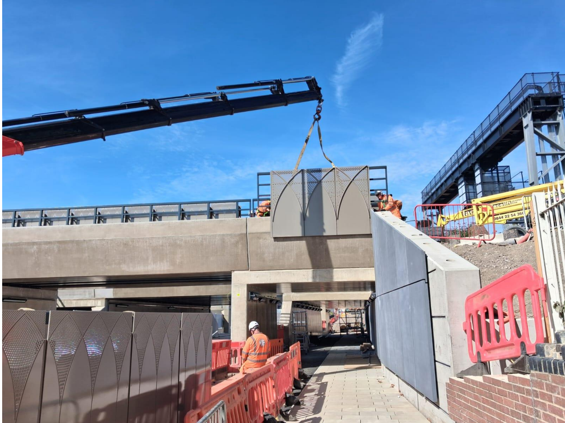
Above: Architectural panels for bridge parapets being installed on east bridge span
