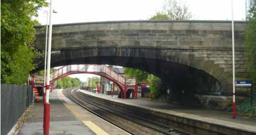
Aberford Road (HUL4/18)
