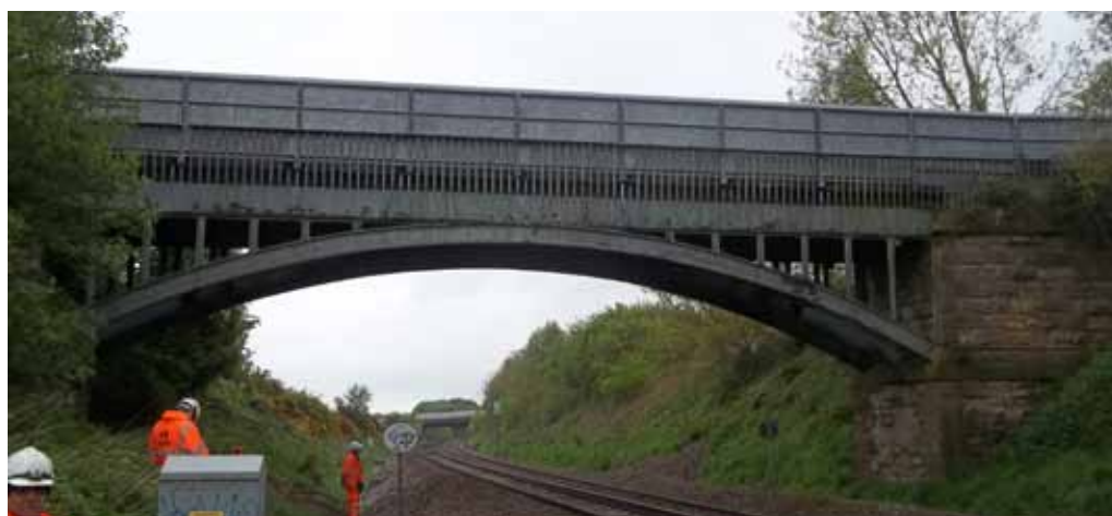
Crawshaw Woods bridge (HUL4/20)
