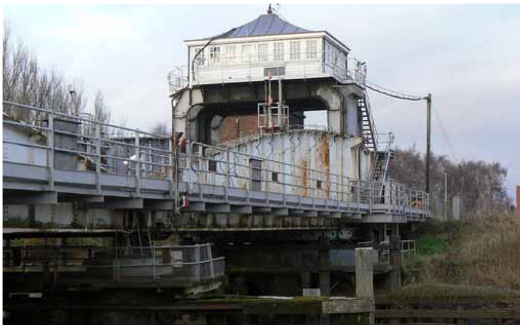
The 1888 swing bridge at Selby
