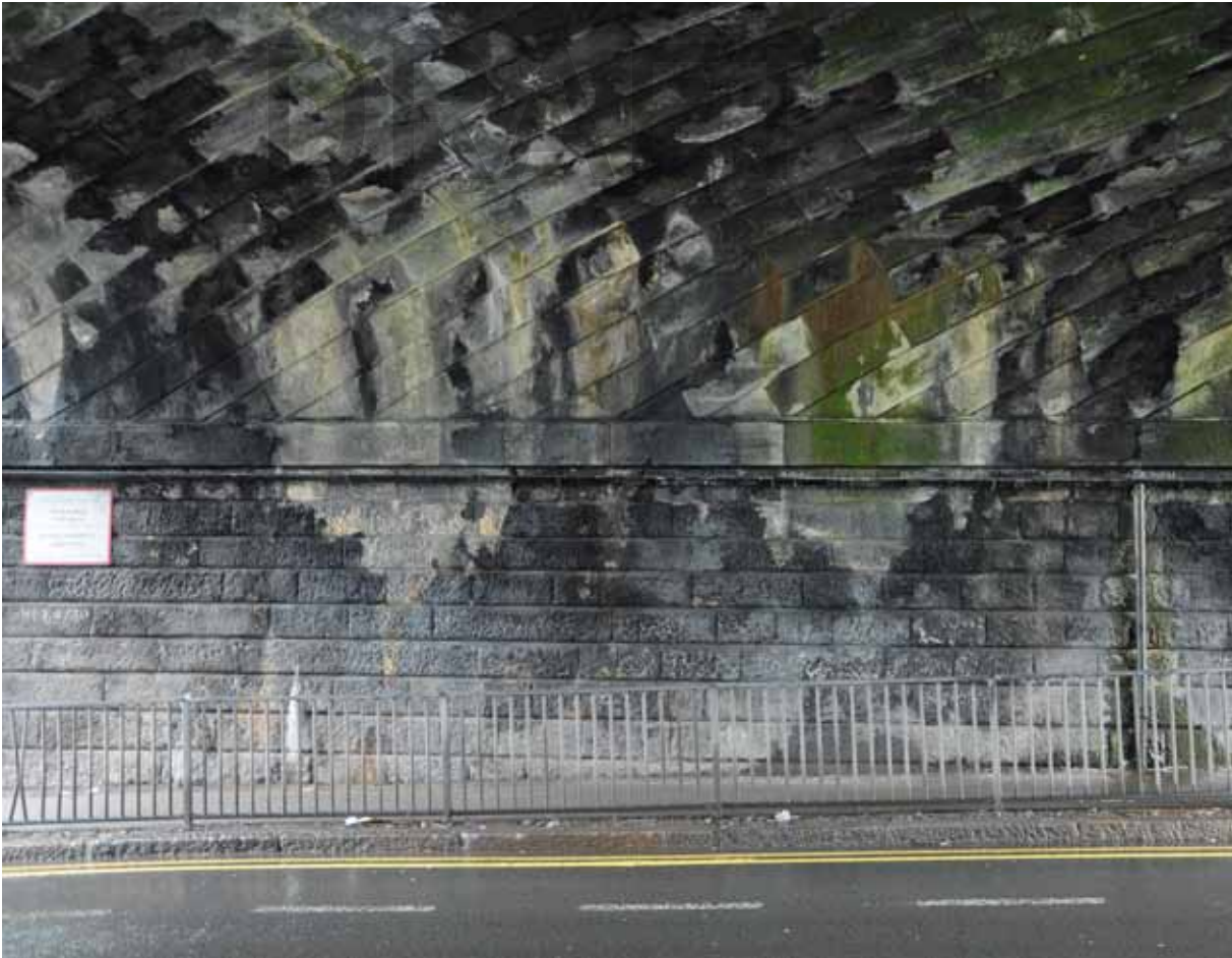
Examples of the outstanding stonework of Leeds & Selby Railway bridges, which were completed in 1834: above, Halton Dial (HUL4/30); opposite top, Roman Ridge Road (HUL4/14); opposite below, Austhorpe Lane (HUL4/21)
