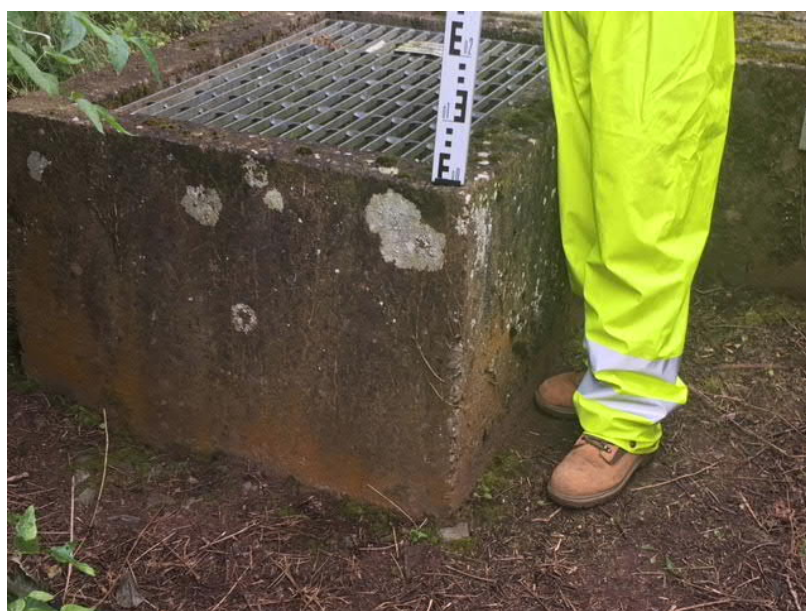
Figure 6-15 – Top of concrete to sewage treatment plant outlet pipe surround
