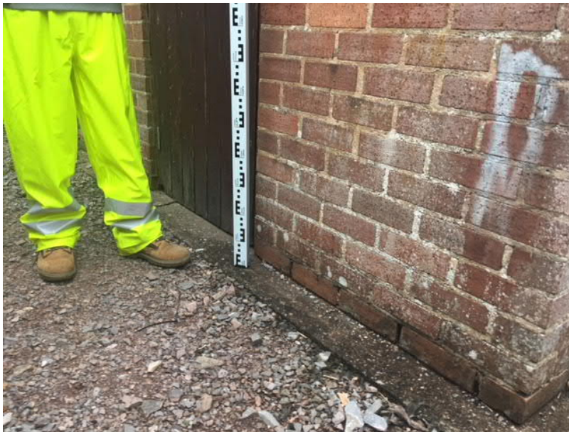
Figure 6-16 – Pumping Station threshold
