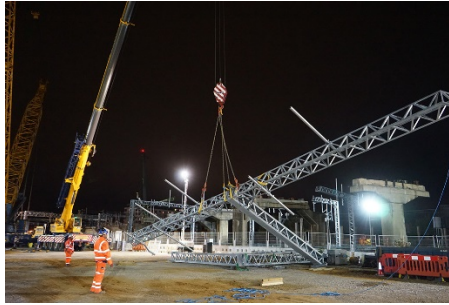
New Overhead Line Equipment (OLE) is installed
