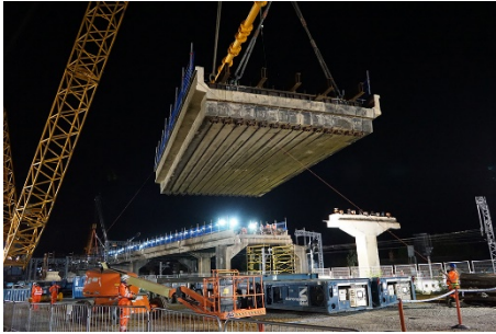
A span is lifted from Bletchley Flyover
