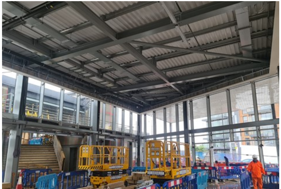
Installation of lighting inside new Hayes & Harlington building
